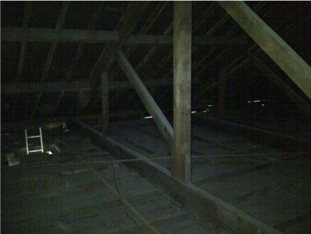
Main chapel roof space
