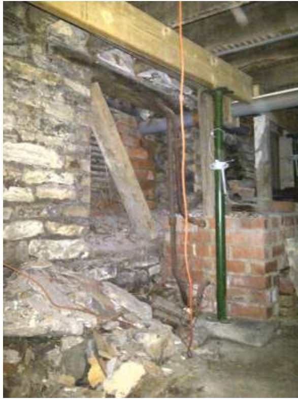
Propping of floor over kitchen
