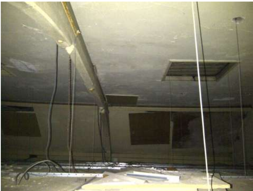
Ceiling area above the suspended ceiling in the meeting room.
