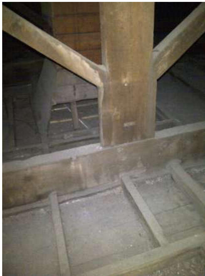
King truss and floor noggins over main chapel
