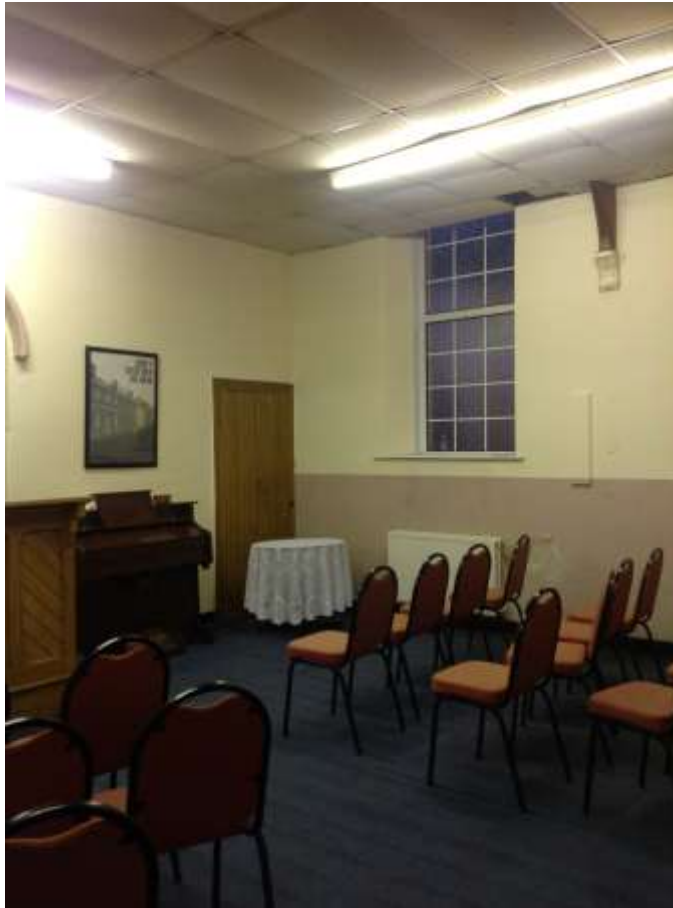
Suspended ceiling tiles over meeting room.
