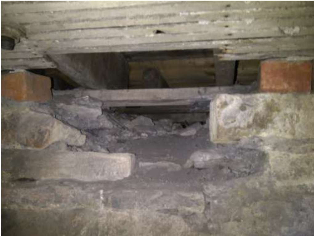
Floor void under meeting room.
