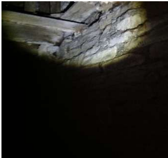
Defective joists over sanctuary (Southern end)
